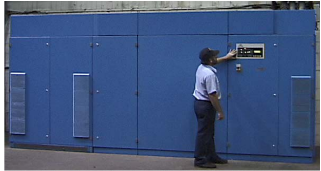
Fig. 7. The 1000 kVA flywheel based UPS.
