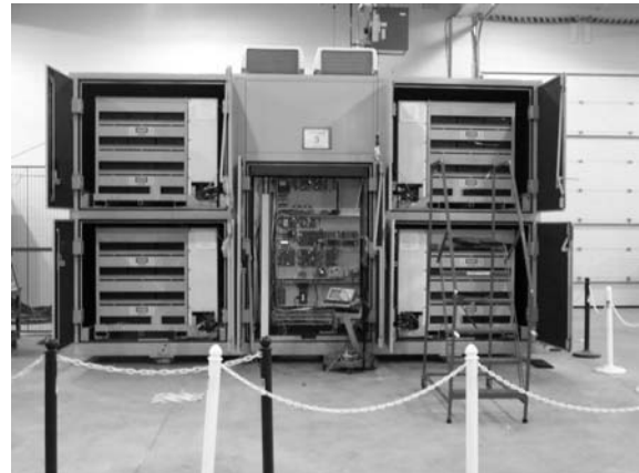
Fig. 3 – Outdoor 2.5 MVA UPS Container
