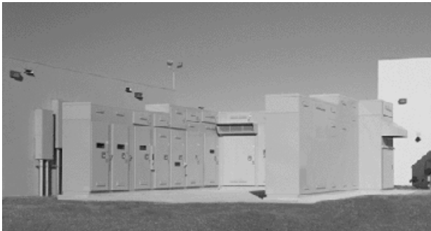
Fig. 7 – Typical Medium Voltage High Speed Static Transfer System at a Semiconductor Wafer FAB
