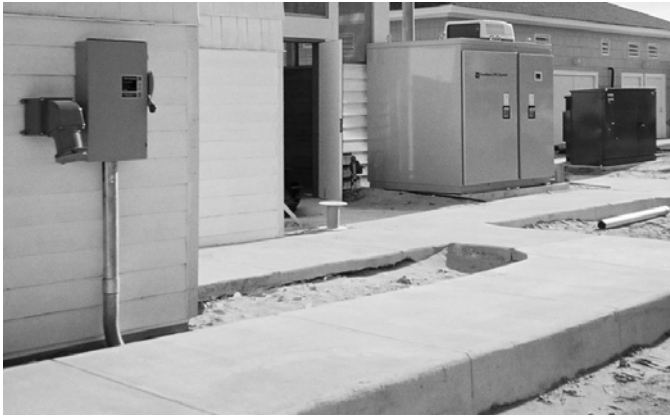
Fig. 4 – Typical Outdoor UPS Installation at a Hospital
