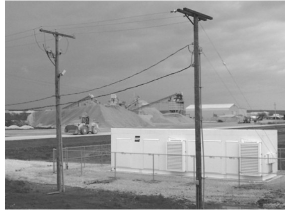
Fig. 11 – DSTATCOM Installation at Rock Crusher Installation
