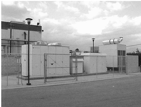
Fig. 5 – Outdoor UPS with Back-Up Generator
